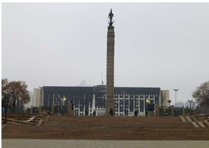
Almaty Akimat Building. Via Wikimedia .
